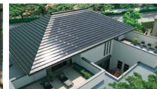
Sekisui House proprietary tile-shaped photovoltaic panels
