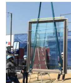
The SHAWOOD large-scale fixed sash combined construction method
