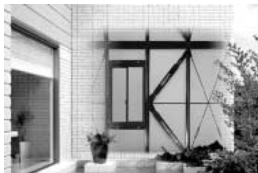
"SHEQAS" Seismic damping system
