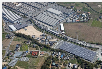
Yamaguchi Factory mega solar
