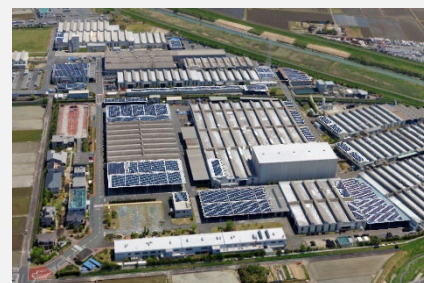
Shizuoka Factory mega solar
