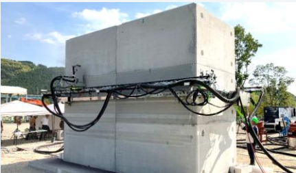
Construction automation using robots (Surface treatment work for seismic reinforcement of bridge piers)
