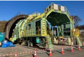
Tunnel lining rehabilitation method “Relining method”
