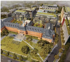
CityRidge Roadside project
