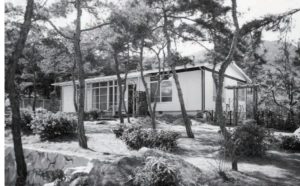
Launched Model B, the origin of our mainstay products, in 1961 Began designing gable roofs and using A panels, high-performance factory-produced exterior aluminum sandwich panels
