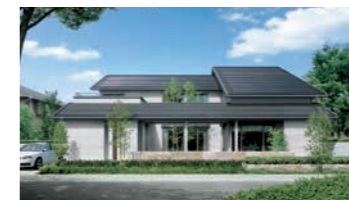
Green First Zero, a net zero energy house that provides comfortable living while reducing CO 2 emissions through the use of photovoltaic power generation
