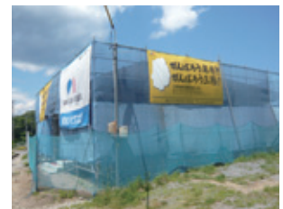
A “Ganbaro Tohoku” house under construction in the stricken area
