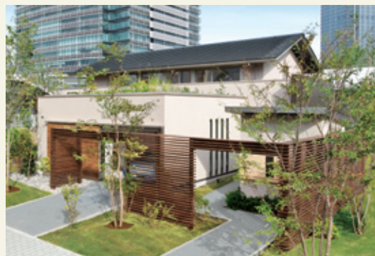
Demonstrative experiments were conducted in the Kankan kyo prototype smart house (in Yokohama City) to develop an ideal future housing environment combined with an electric vehicle. (2010)
