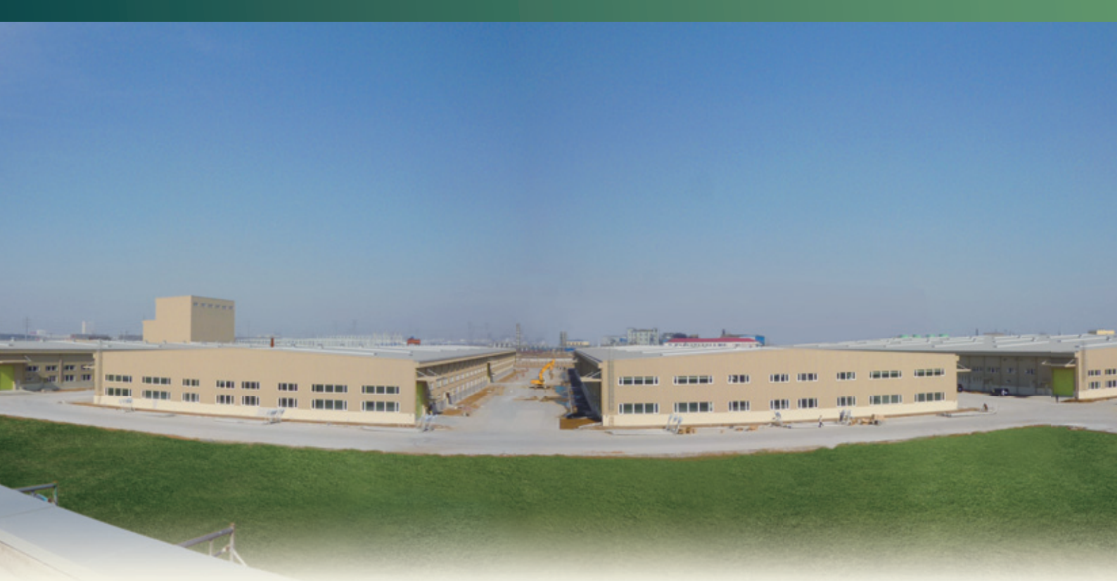
Sekisui House is the first to start production using a Japanese industrialized housing system in China.
