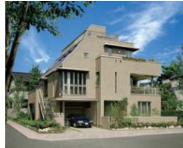
"BIENA" three-story steel-frame detached house
