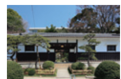
Emphasis placed on creating a balance with the beautiful local natural environment and preserving the existing structure during the construction of the condominium
