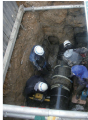
Recovery work continued all-out amid repeated aftershocks.
