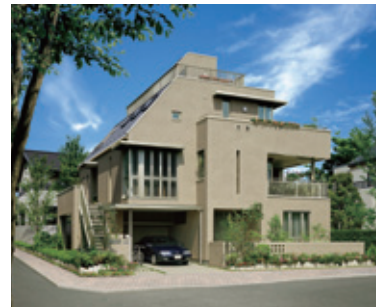
"BIENA" three-story steel-frame detached house
