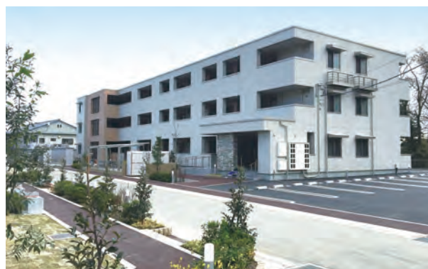
Disaster-ready public housing in the Kujo district of Kesenuma, Miyagi Prefecture (completed in November 2016)
