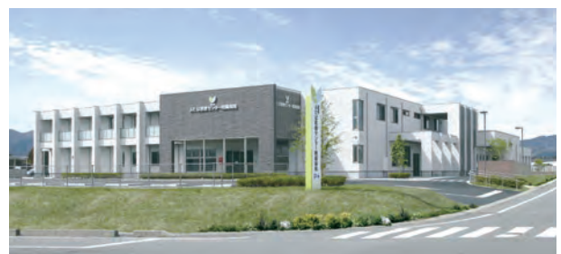
Hospital constructed with the Flexible \beta System (Futaba Medical Center, Fukushima Prefecture)
