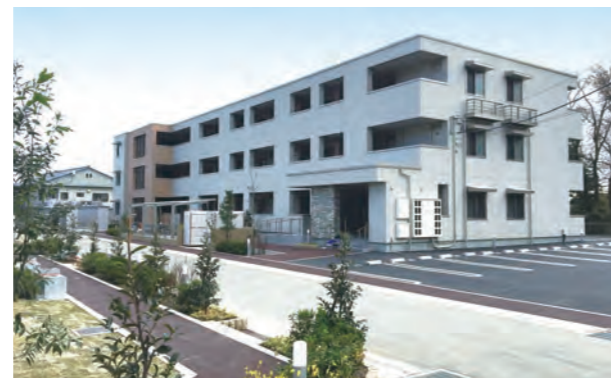
Disaster-ready public housing in the Kujo district of Kesenuma, Miyagi Prefecture (completed in November 2016)
