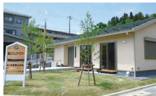
Disaster-ready public housing in the Tateyama district of Kesenuma, Miyagi Prefecture (completed in May 2016)
