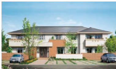
Installed PV systems on Sha Maison apartments and remodeled houses with new insulation
