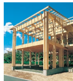
Wooden rigid-frame construction allows house designs with wide openings on three sides and a large built-in garage
