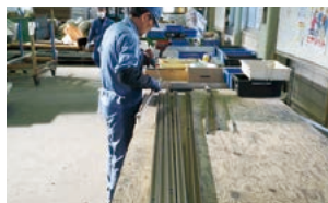
Dismantling window sashes into metal and glass parts
