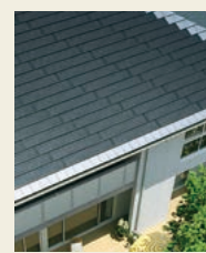
Roof tile-integrated solar panels
