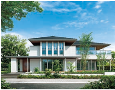
Is Roy+E two-story steel-frame detached house
