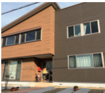
Children's Development Support Center, built based on Sekisui House's SHAWOOD design for wooden-frame houses
