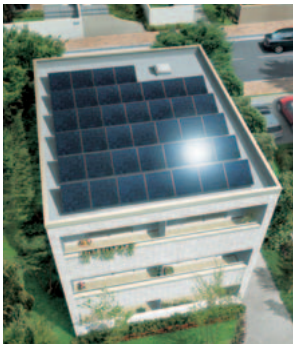
Fixed-installation solar panels
