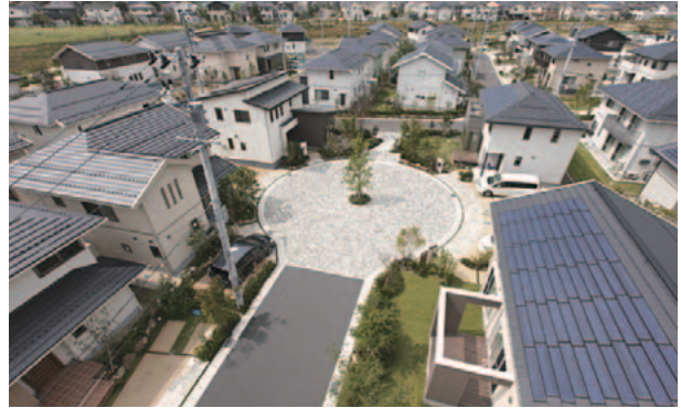
Green First HYBRID homes, which employ three types of power supply cells, surround the cul-de-sac. Even during a blackout, this space can be lit up. In times of emergency, the open space serves as an evacuation site for residents.
