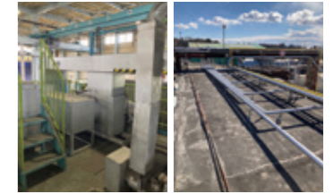
Change of the heat source for drying furnaces from boiler heat to burners
