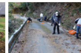
Removing dirt from landslides (November 27)
