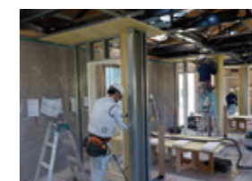
Interior finishing course: completion test
