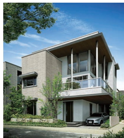
Both the open balcony space and the installation of high-capacity solar panels are made possible with columns that support the large roof on the second floor.
