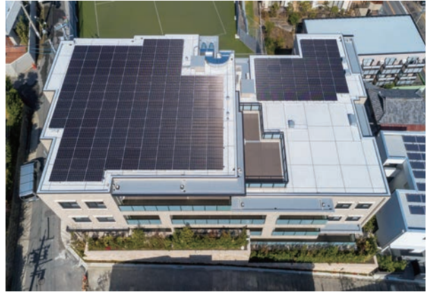
Grande Maison Kakuouzan Kikuzakacho in Nagoya, a low-rise condominium complex (All units are ZEH.)
