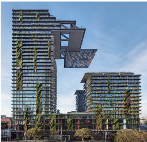
Aerial gardens, impressive green walls, and reflectors to take advantage of natural light
