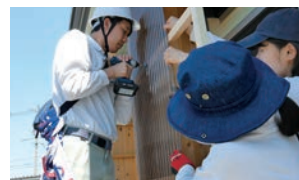
Windbreak wall installation on temporary housing
