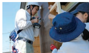
Windbreak wall installation on temporary housing
