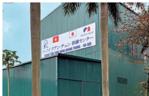
Technical training center in Hanoi, Vietnam (exterior)
