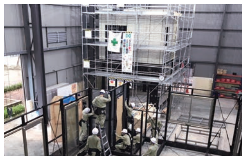
Exterior frame building exercise in Hanoi, Vietnam
