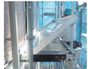
AS Balcony, a "physical resources" solution
