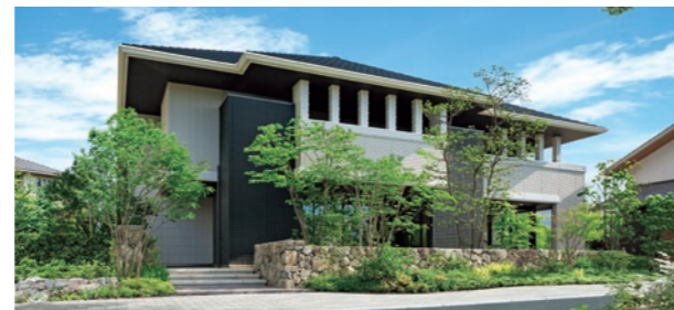
IS ROY+E steel-framed two-story house
