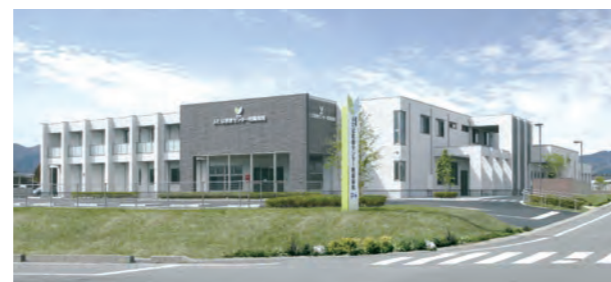
Hospital constructed with the Flexible B System (Futaba Medical Center, Fukushima Prefecture)
