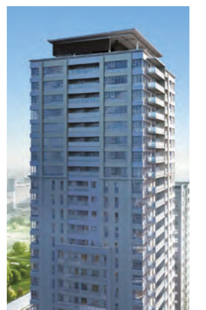
Grande Maison Uemachidai The Tower, in which all the units are equipped with Ene-Farms.
