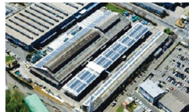
Operated mega-solar power systems at 5 factories for a total of 6.7 MW
