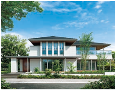
Is Roy+E two-story steel-frame detached house
