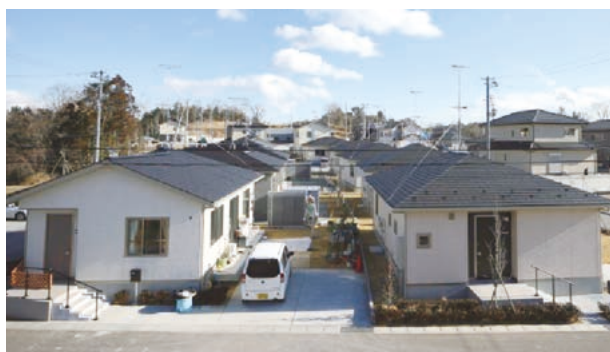
Public housing in Shinchi Town, Fukushima Prefecture
