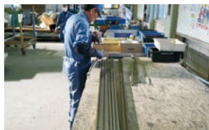
Dismantling window sashes into metal and glass parts
