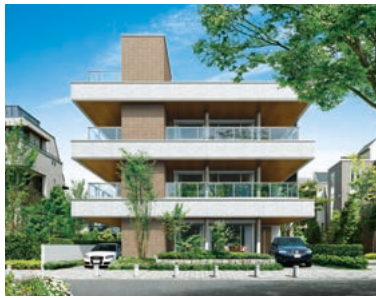
Bienna three-story steel-frame detached house
