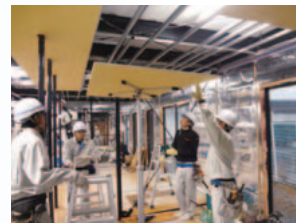
On-site training for installing plasterboard on ceilings
