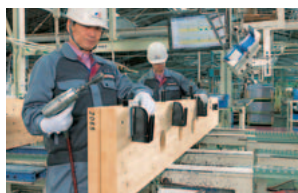
Metal fittings are pre-attached to structural frames to reduce the workload at construction sites
