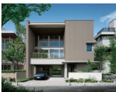
Biena three-story steel-frame detached house
