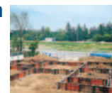
Use of a Metal Form steel frame enables the construction of foundation work with uniform quality and precision, regardless of the workers' skill level
