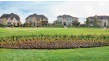
Cinco Ranch in Texas, USA
