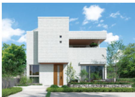
“IS ROY+E”: Luxury Modern Series, two-story steel-frame detached house
