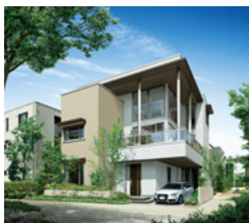
“BIENA” three-story steel-frame detached house
