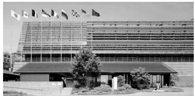
The introduction of Japanese advanced environmental technologies to interior/exterior parties in front of the International Media Center during the G8 Hokkaido Toyako Summit
