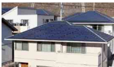
Roof tile photovoltaic power generation system designed to harmonize with the surrounding townscape
