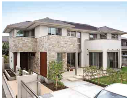
The house is provided with a 5.2 kW PV system.
