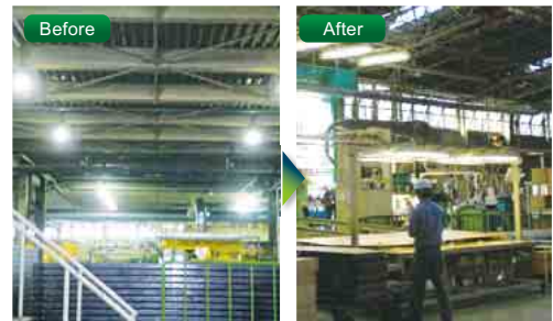
Mercury lamps for general lighting were replaced with fluorescent lamps for close lighting.
