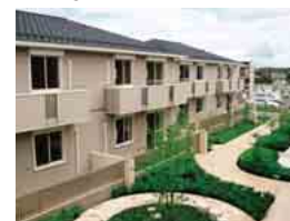
Terrace-style Sha-Maison Green First apartment. Each residential unit (79.5 m 2 ) consists of three rooms and a living-dining room plus kitchen, and a 2.2 kW PV system is provided in each household.
