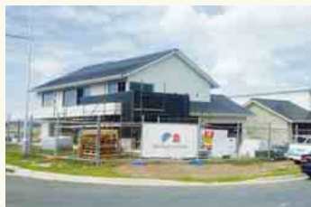
A display home equipped with a roof tile photovoltaic power generation system
