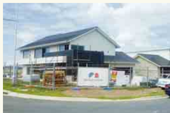
A display home equipped with a roof tile photovoltaic power generation system
