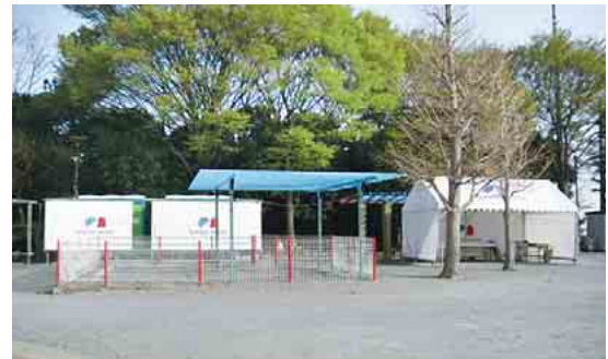
A temporary lavatory is installed in an open space in the residential estate we developed.
