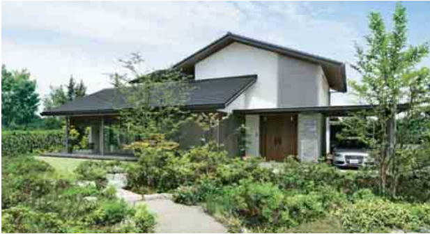
BeSai+e steel-frame detached house
