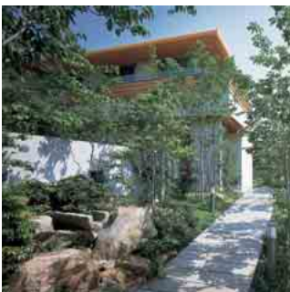
Exterior construction work
