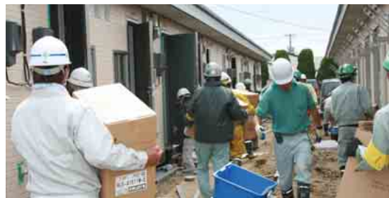
Many construction personnel are mobilized from all over Japan to work in the stricken areas.
