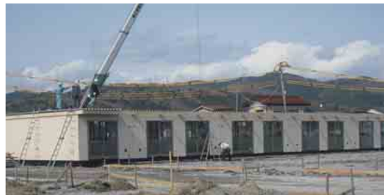
Temporary houses are built at an accelerated pace.
