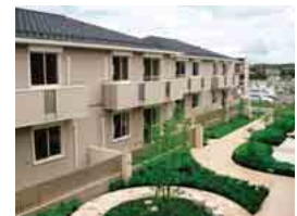
Terrace-style Sha-Maison Green First apartment. Each residential unit (79.5 m 2 ) consists of three rooms and a living-dining room plus kitchen, and a 2.2 kW PV system is provided in each household.
