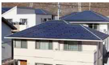
Roof tile photovoltaic power generation system designed to harmonize with the surrounding townscape
