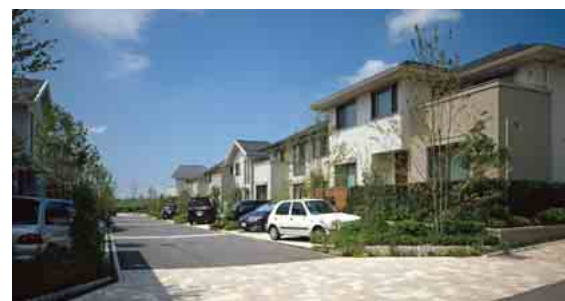
We are developing a community of Chemicare homes in Kazusa no mori Chiharadai (Chiba Prefecture).
