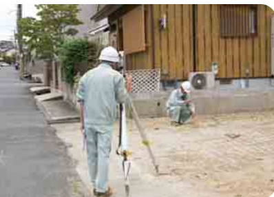
In a site survey, we check the exact gas and water pipe locations.
