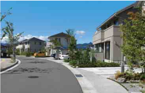
"Common Stage Tenjin no mori," detached houses project
