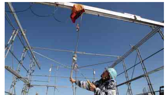
We use our proprietary “girder crane” system on the construction site. We conduct frame construction and exterior work using an overhead crane that is temporarily installed on the upper part of scaffolding.
